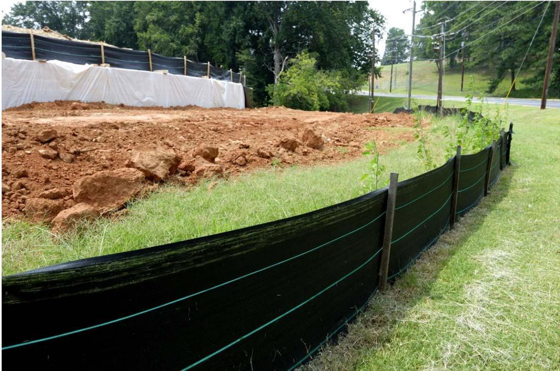
Figure 5.3 Example of Silt Fencing
