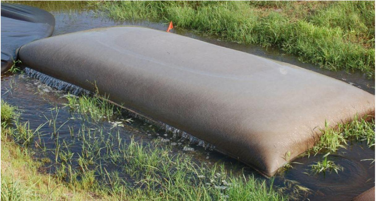
Figure 5.4 Example of Silt Dewatering Bag
